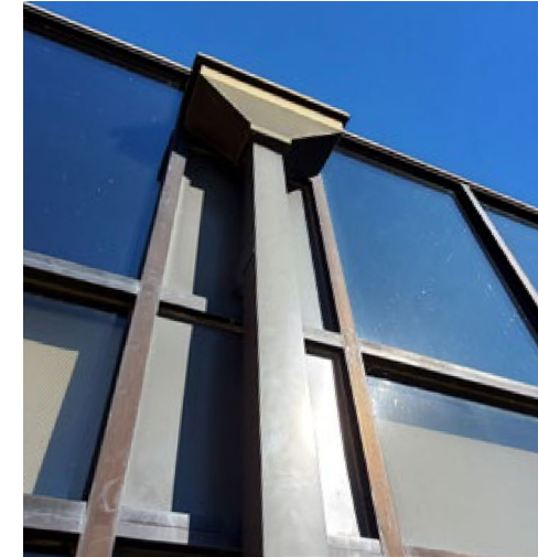
Scupper and Downspout
