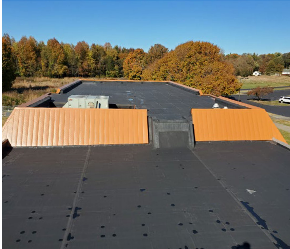
Roof Looking West
