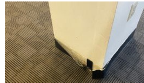
Damaged Interior Finishes
