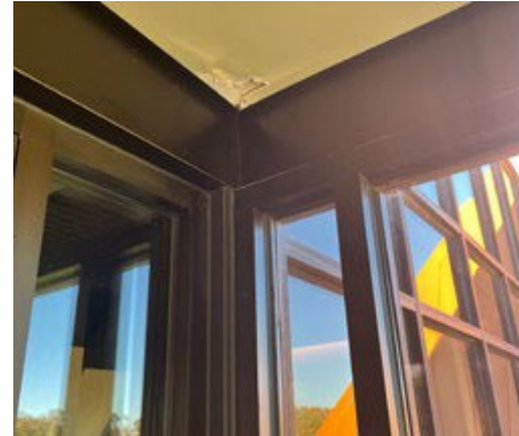
Main Entry Vestibule Ceiling Condition
