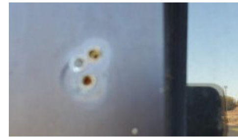
Penetrations in Storefront
