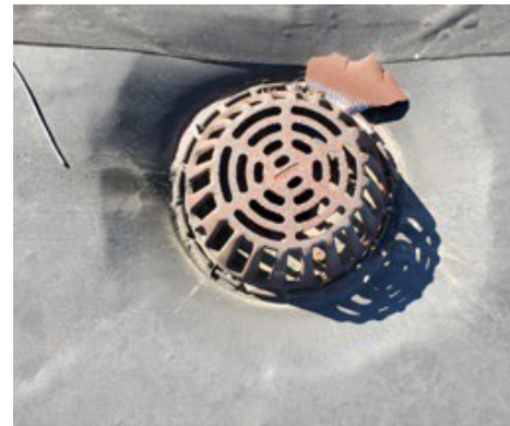
Typical Roof Drain
