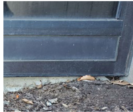
Deteriorated Concrete at Grade
