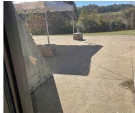
Exterior Amenity Space
