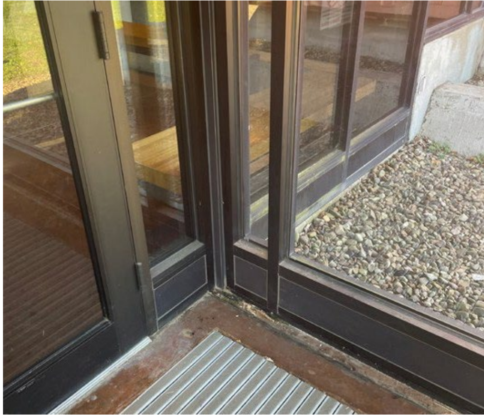
Main Entry Vestibule Floor Condition
