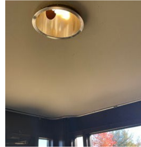
Main Entry Vestibule Lighting
